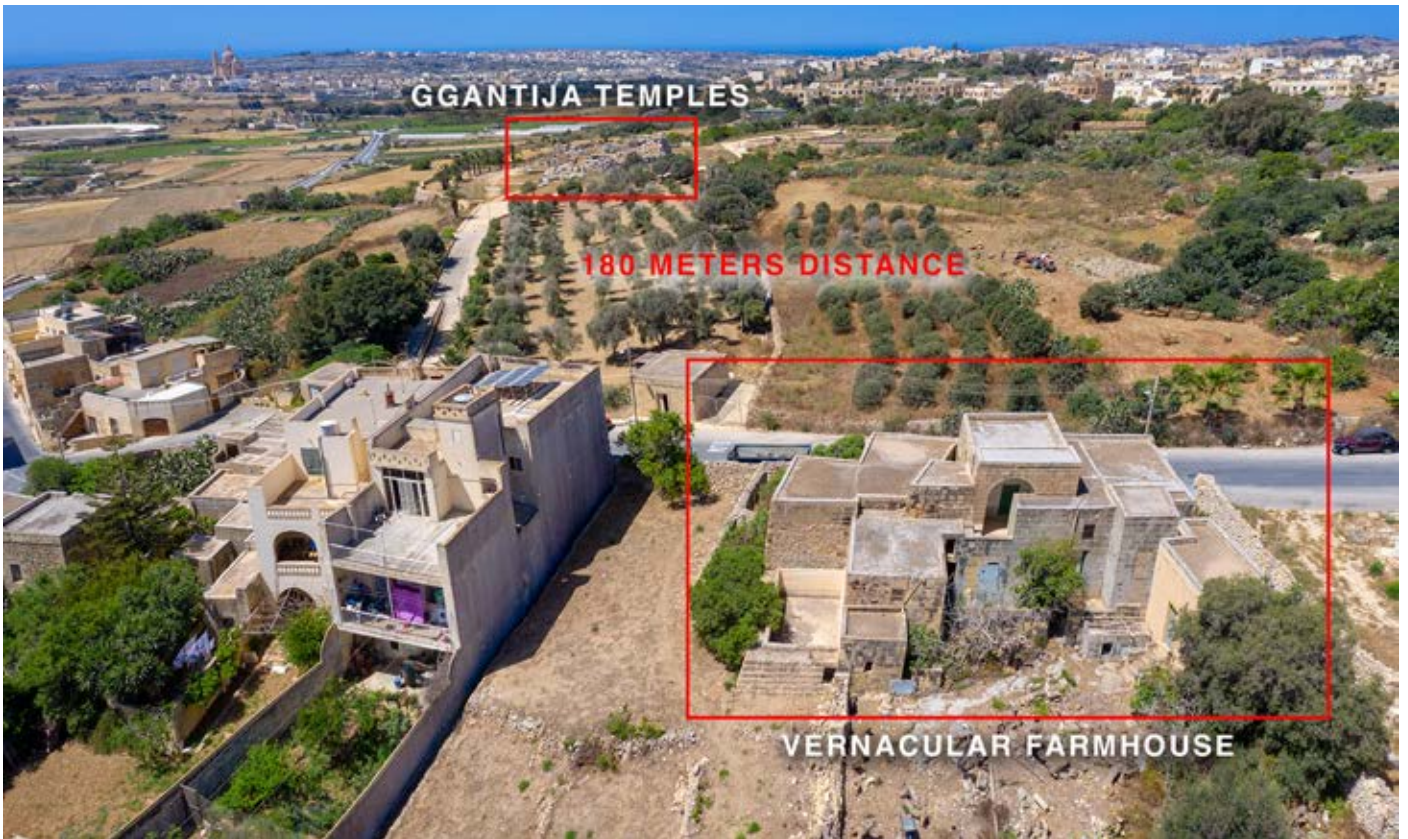
Figure 6. The vernacular farmhouse earmarked for demolition lies in close proximity to the Ġgantija Temples.
