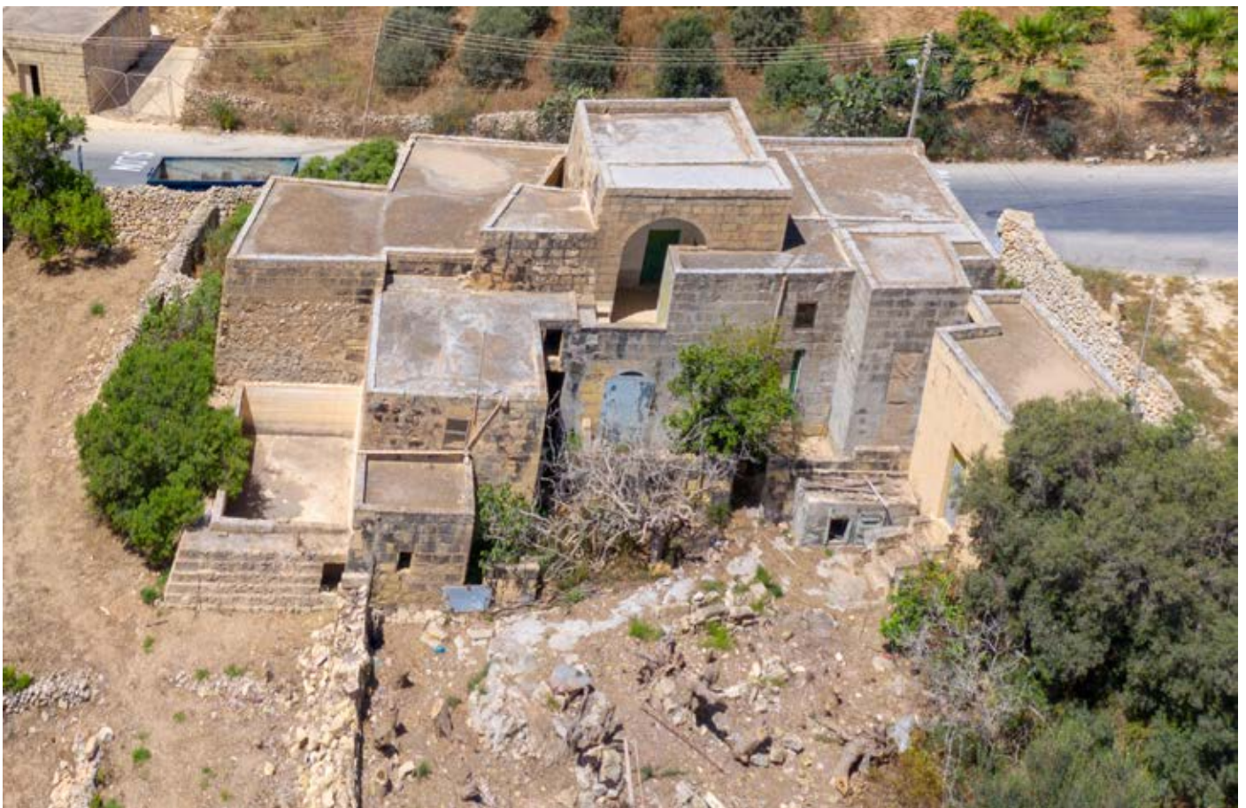
Figure 7. The vernacular farmhouse that is to be demolished to make way for the new development. Parts of the building are of considerable age, as rubble masonry was used in its construction (see IHA 2244c, page 52 (page 62 of 85 of the PDF), Plate 16. The farmhouse incorporates above-ground and underground water reservoirs, living quarters and animal sheds within the same structure.
